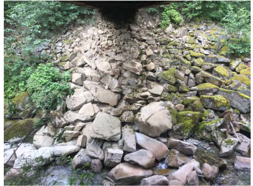
Right Bank Abutment when facing downstream
