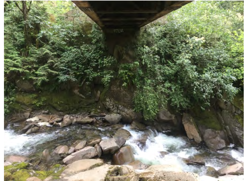
Left Bank Abutment when facing downstream
